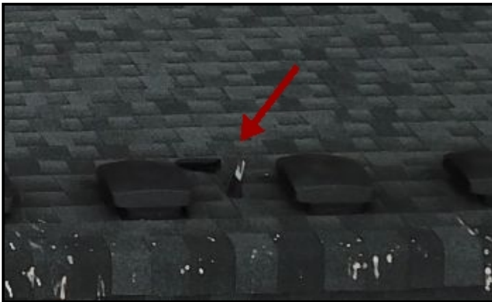
Roof anchors covers are not in place. This can lead to rust on the anchors. Recommend roof anchor covers are placed over anchors.
