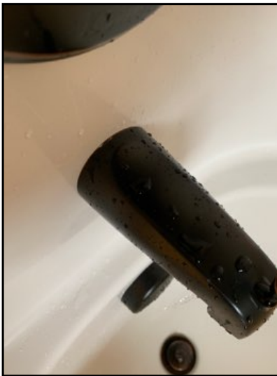
Caulk at base of tub spout.
