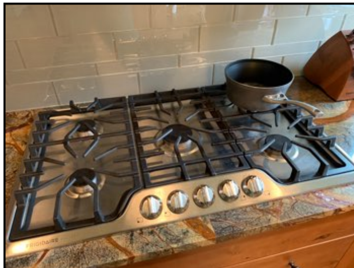
Gas cook top noted.
