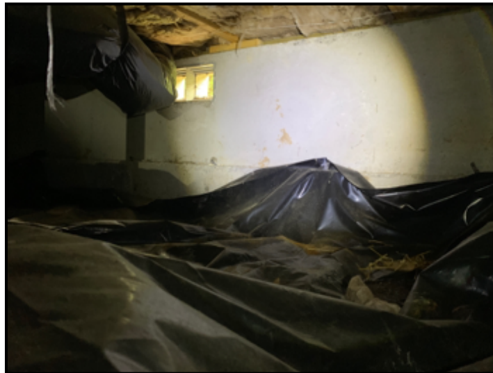
Walls appear functional.
