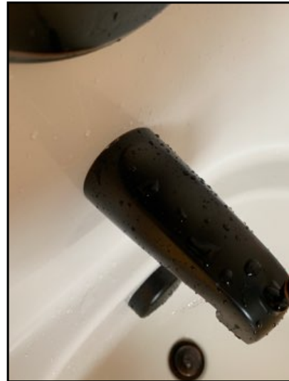
Caulk at base of tub spout.
